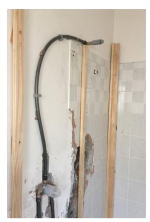
Tiling was too uneven and unstable to have the Fibo panel fixed directly with adhesive over the existing tiles. Instead, the wall was battened out and aligned using packers. The Fibo distributor assisted by surveying the room and preparing a framing plan with take-off. battens set at 600 centres to be in line with panel widths. Panels are fixed with a screw through the groove, a modern form of secret nails.
